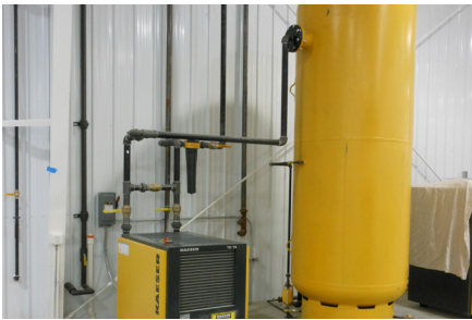
Simply connect the CA to existing plant air or a centralized compressor.
